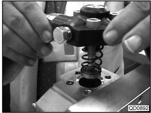
(10) Pull the element sub-assembly until it faces straight up and remove the element sub-assembly, plunger, and spring in the same way as step (5).
